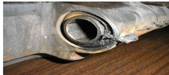
a) Bushing/Track Block Failure – Bradley T-157
